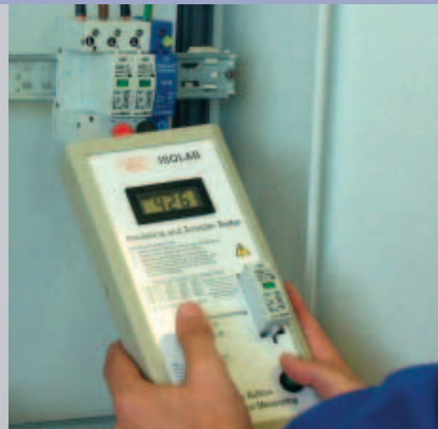
Measuring surge arresters
